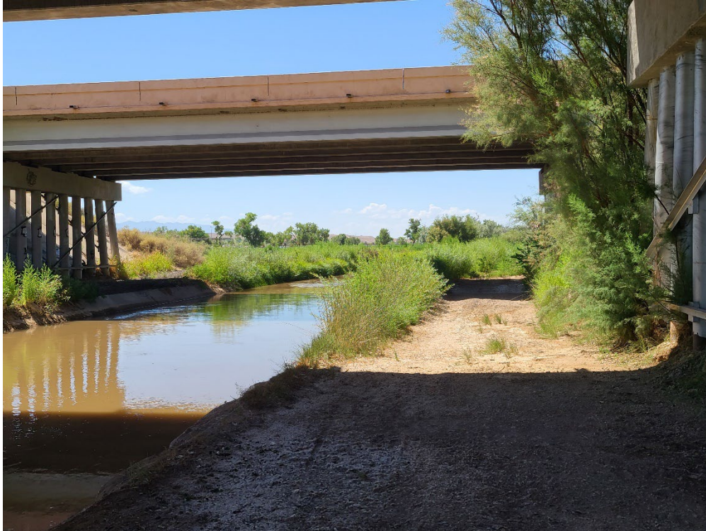
Section of cement-lined Albuquerque Riverside Drain under the I-25 bridge
