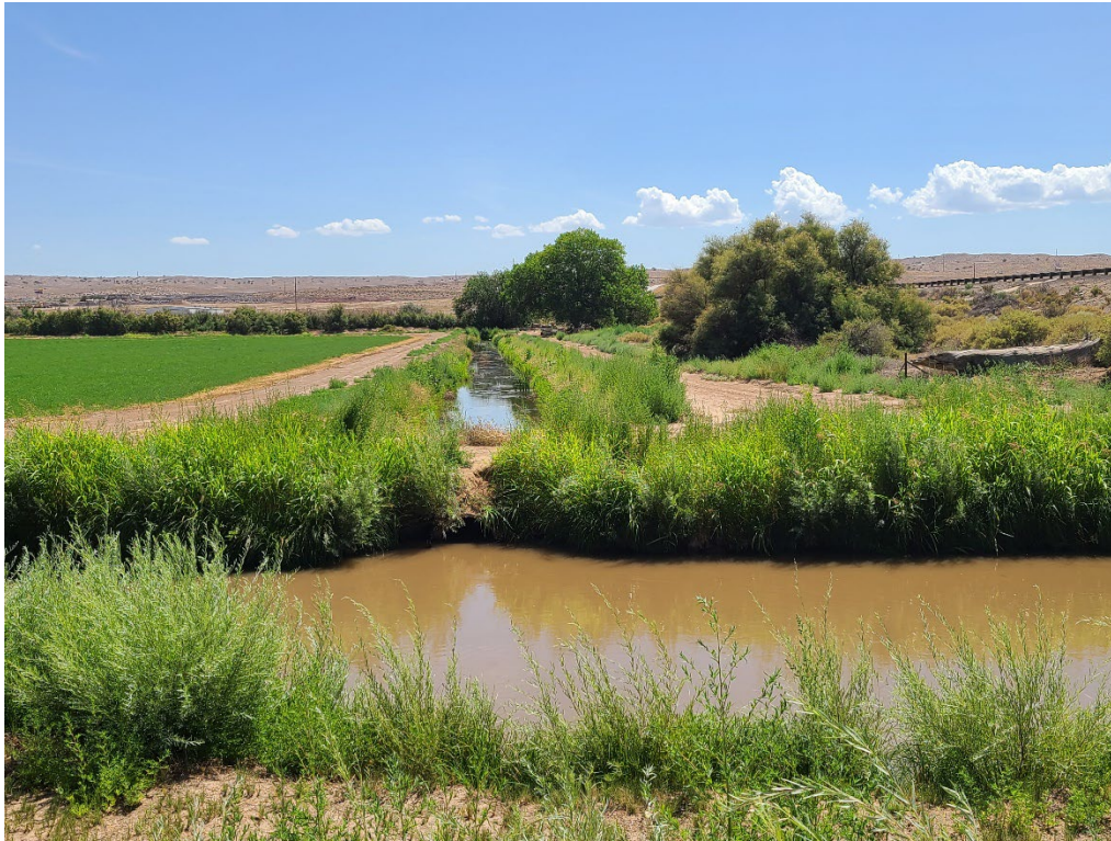
Intersection of the Barr Lateral Ditch with the Albuquerque Riverside Drain.
