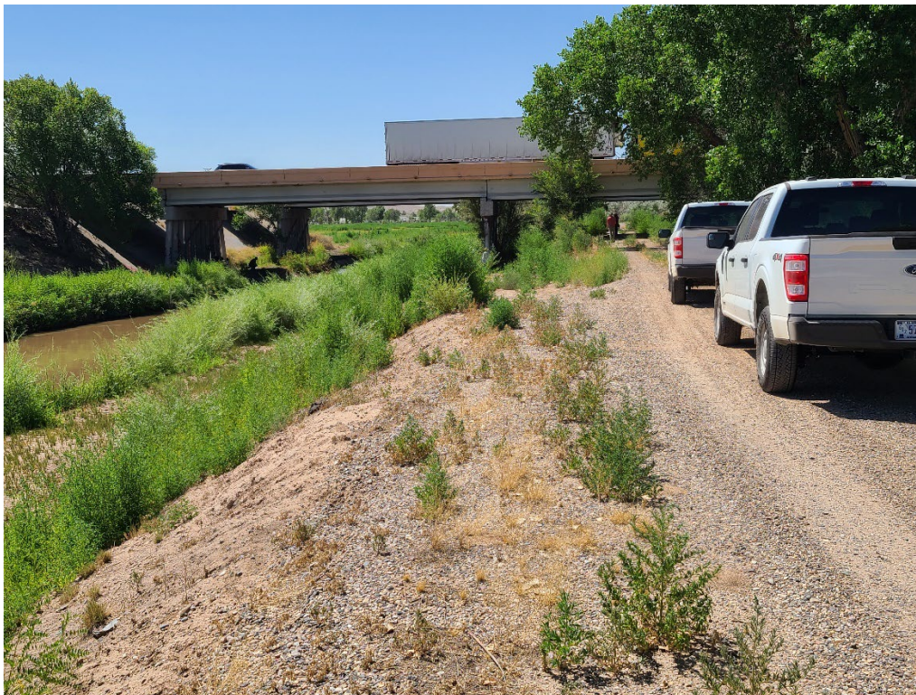
Trucks parked on the existing Spoil bank levee next to the Albuquerque Riverside Drain between the proposed culvert location and the I-25 bridge.
